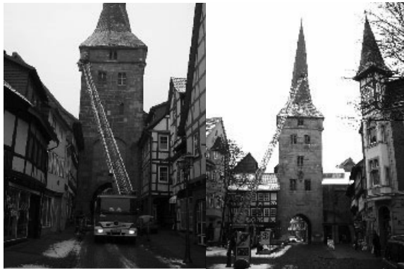
Figure 4: Mobile turning ladder at the West Tower in Duderstadt for signalling of control points and for image recording
