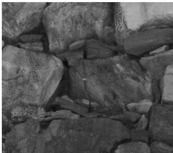
Figure 2: Laser on a control point
