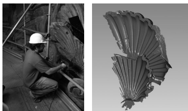
Figure 12: Survey of the stone decorative elements of the Guarini Chapel on a scaffold and 3D model
