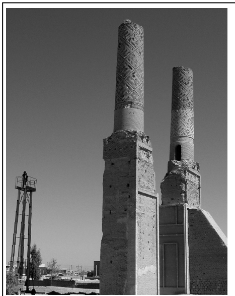
Figure 6: Documenting inaccessible parts using a lift
